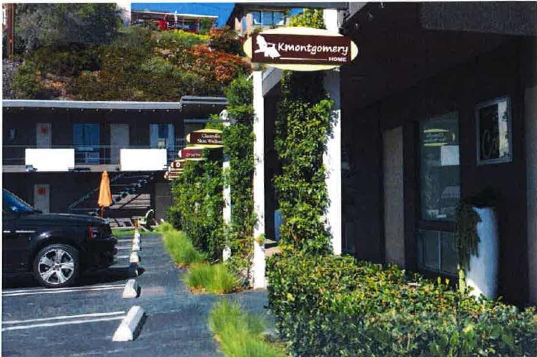
PHOTOGRAPH 4 – View looking north at the east wing of the Shops at the Cove at 410 West Coast Highway. The two-story wing is at the rear of the parking lot. A residence is seen at the top of the slope north of the Site.
